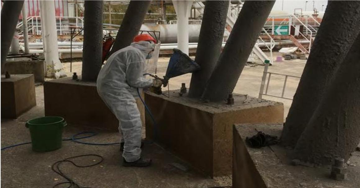
**Figure 126.** Spray-coating the GF on the surface of the pillars by the thesis author.
