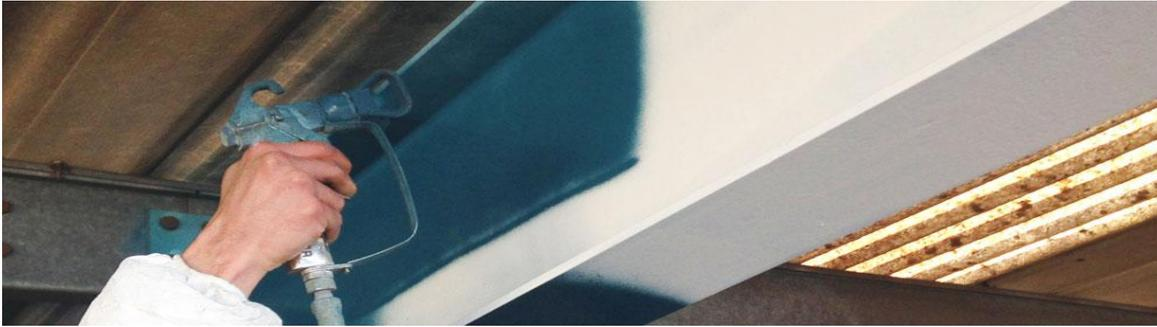
**Figure 5.** Fire-resistant paint for steel [19].
